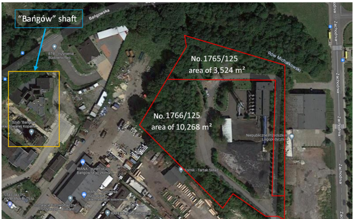
Figure 35. Location of the facilities in the area of Siemianowice Śląskie 36
